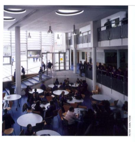
11. The roof is 'peeled back' to form rooflights
