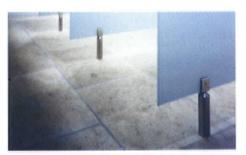
CNC turned stainless steel feet. Bolted into the floor and set out of sight 200mm, back from front of cubicle.
