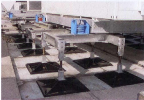
supports Part L regulations for air tight and no cold bridging
