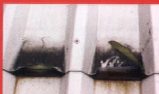
Leathergrain plastisol roof after 7 years
