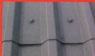
Colorcoat HPS200® roof after 7 years
