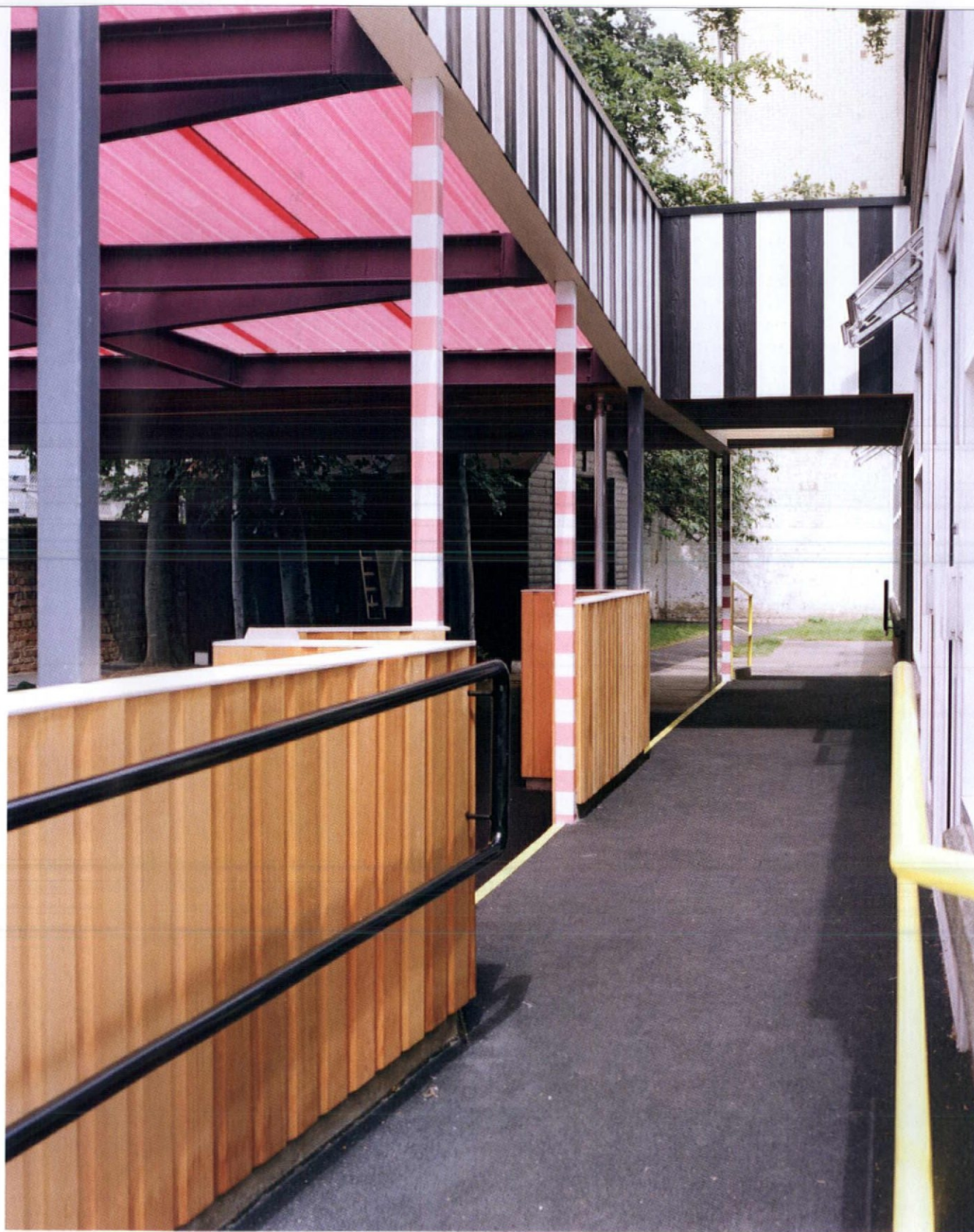
19. The steel joists zig-zag playfully as they support the pink GRP and its black-and-white bargeboards
