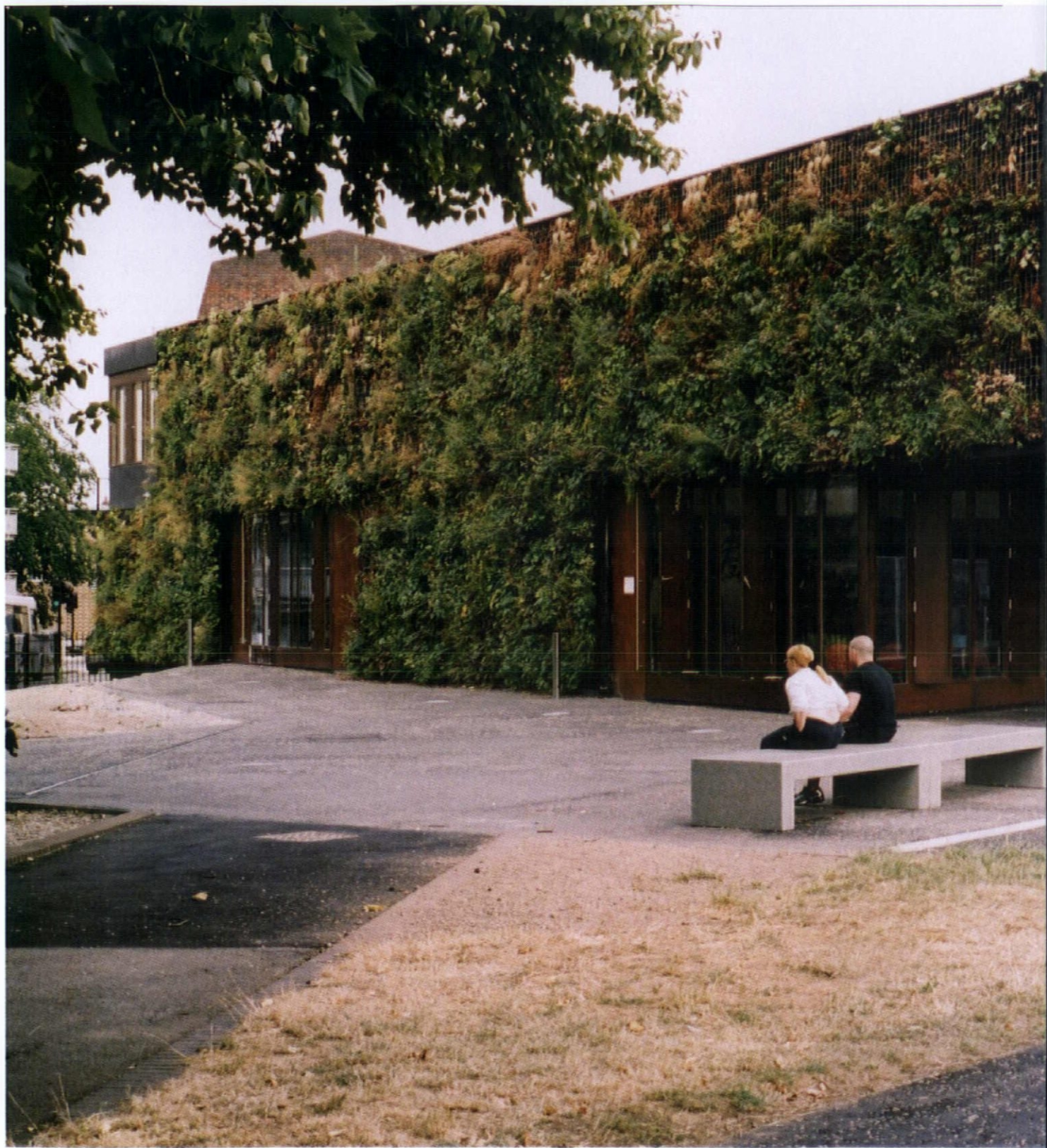
13. Steel mesh cases, filled with growing medium, are bolted to the facade to create the green wall
