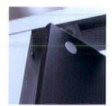
12mm solid grade panels, polished on all edges, through fixed to aluminium frame.
