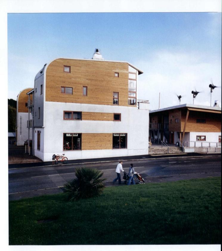
5. The lower down-wind block is designed to lift the wind up and over itself, the court and the taller block without turbulence
