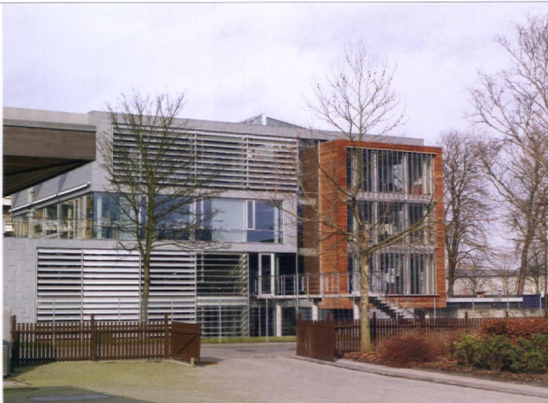
1. Southern elevation: a continuous zinc-clad ribbon rises from the ground to crank around the top two floors
