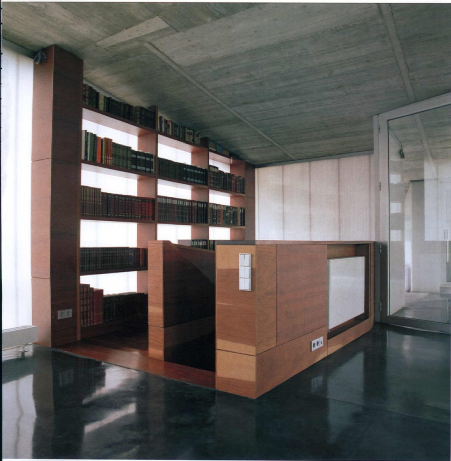
16. The lounge has a shuttered concrete ceiling and black pigmented concrete floor
