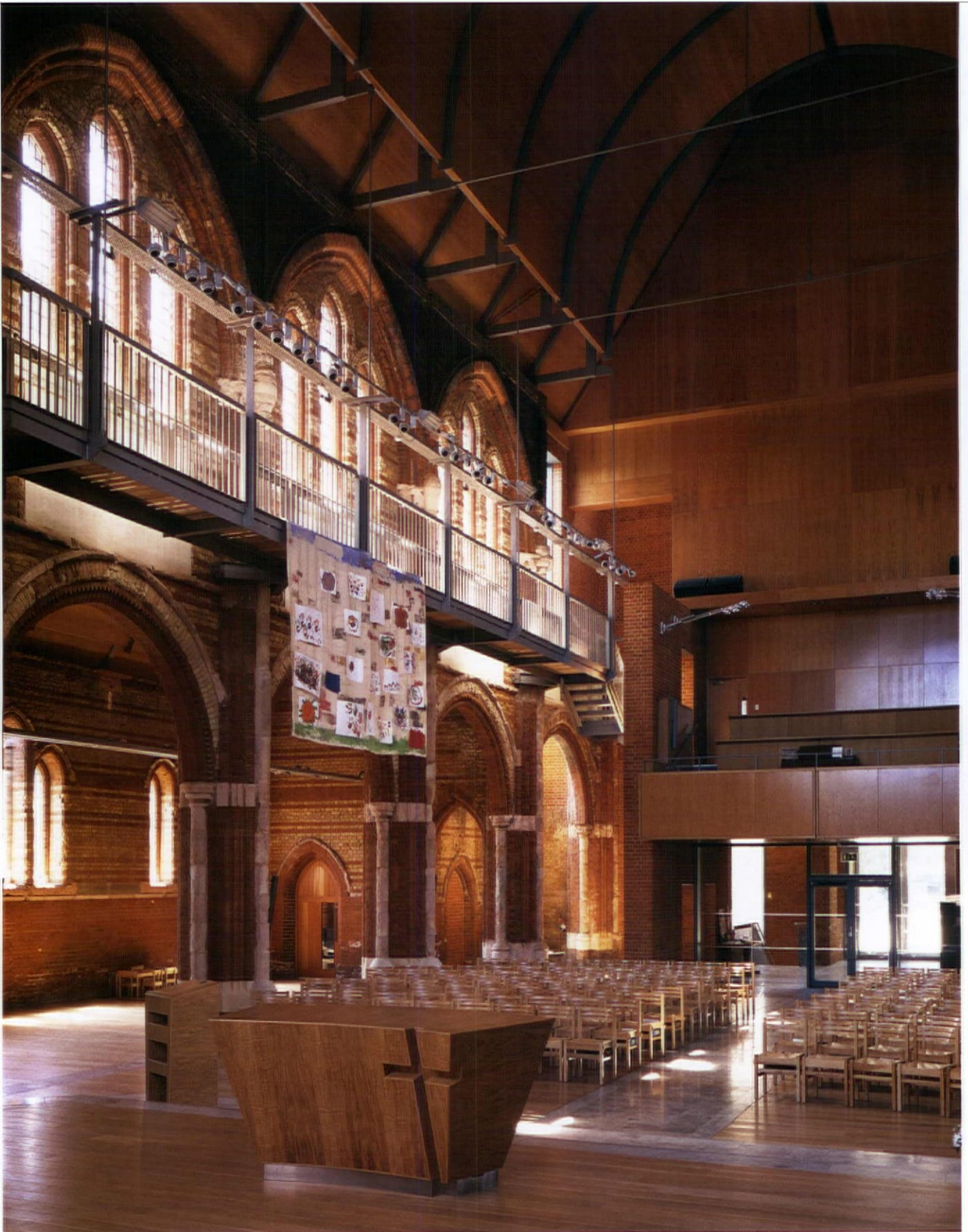
6. A new access and lighting gantry forms a gallery above the nave arcade
