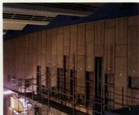
Panelling removed and refitted
