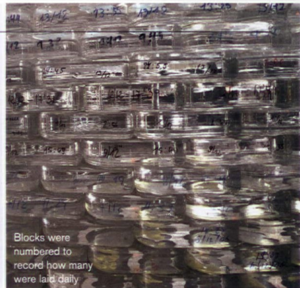
Bespoke blocks of moulded borosilicate measure 200 x 300mm and are 70mm thick
