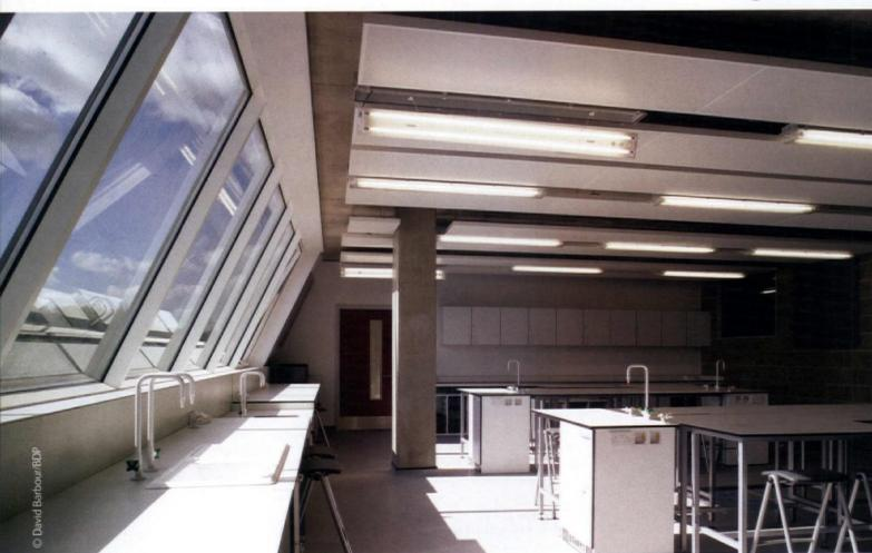
At Grace Academy, Solihull architects BDP required a **robust** solution which met the demands for **acoustic performance**. SAS System 600 metal acoustic lighting rafts allow free air movement to the exposed concrete soffit for **sustainable natural mass cooling** whilst achieving acoustic absorption.
