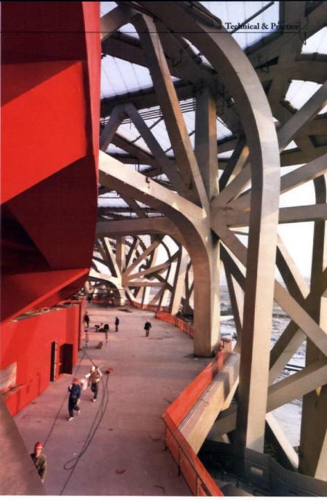
The tangle of steel on the exterior of Herzog & de Meuron's (HdM's) Beijing National Stadium which gives it its distinctive appearance – and the nickname Bird's Nest – is in fact three interconnected structural systems: a primary structure of supporting columns; a secondary 'cladding' structure, which stiffens the columns; and the tertiary stair structures. 'The facade is not a facade, it's a structural grid,' says HdM's Jacques Herzog; 'it is
