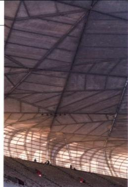
Left Concrete seating bowl with ETFE enclosure
