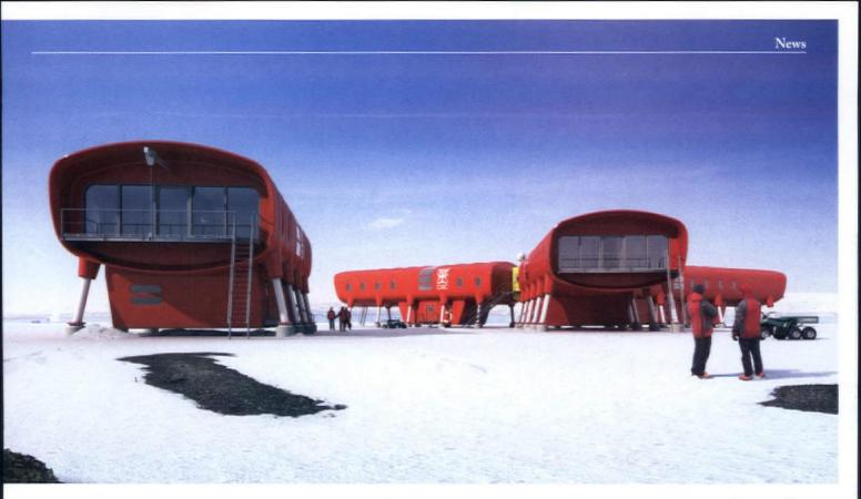
This page The Juan Carlos 1 research station will be constructed from modular fibrereinforced plastic monocoque rings
