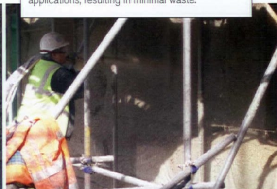
Hemp, sourced from Essex, and lime are mixed on site and sprayed to the building exterior. Excess material is raked off and reused in subsequent applications, resulting in minimal waste.
