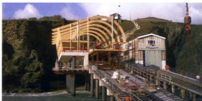
Right A laminated wood-barrel skeleton forms the curved roof
