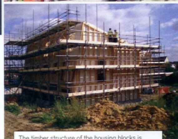
The timber structure of the housing blocks is visible prior to application of Hempcrete insulation, which can be applied in batts or sprayed. A sprayed application results in an airtight construction because the structure becomes embedded in the insulation, minimising the number of joints and optimising the operation of the whole-house ventilation system.
