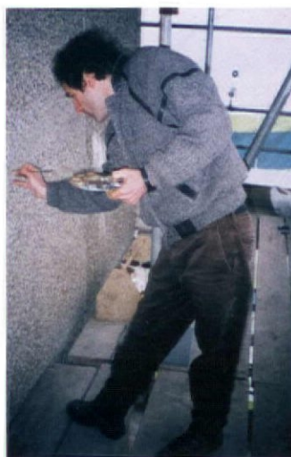
Far left The tonal contrasts of Priory Heights Estate's facade were restored rather than overclad
