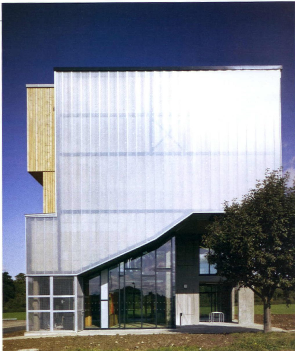
This page The stairs, expressed externally on both the west (left) and south (above) facades, are 'clothed' in a polycarbonate skin' that reveals the centre's structure. The building is entered through the open corner of the east facade, marked by a lime tree (far left)
