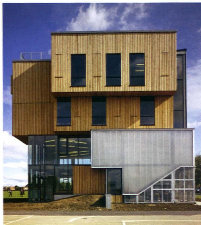
This page The stairs, expressed externally on both the west (left) and south (above) facades, are 'clothed' in a polycarbonate skin' that reveals the centre's structure. The building is entered through the open corner of the east facade, marked by a lime tree (far left)
