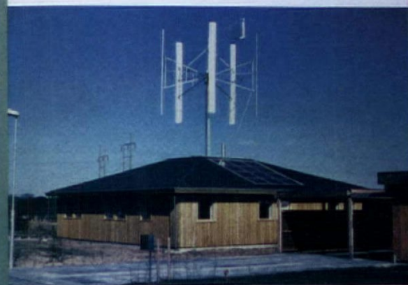
Amongst nine highly different experimental houses in Skive, Denmark, this wind-powered version had a heat-churn system (for creating hot water). It lasted more days when the vibrations were found to be excessive.
