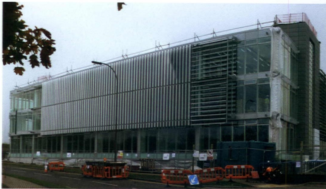
Below West elevation with fixed external louvres for shading Bottom Detail of sunshading fixing to curtain wall
