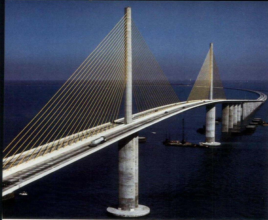
**THE NEW YORK TIMES** stated crossing the main span of the Sunshine Skyway Bridge (left) is almost a religious experience. An aerial view of the structure (below) shows the single row of steel cables that spreads out from the central pylons, which are connected directly to the roadway.
