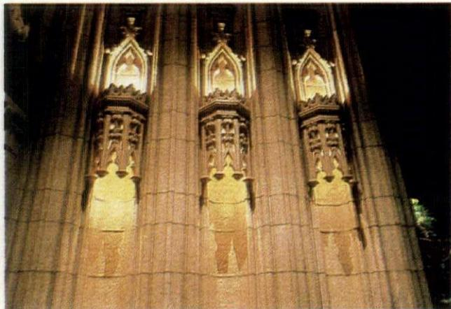
**CLASSIC ARCHITECTURE:** The highly ornamented ceiling (right) houses quartz downlights which provide light for the space below. Illuminating the entry arch are halogen lamps used as uplights behind the sconces (above); halogen lamps also illuminate the pilasters of the building facade (left).
