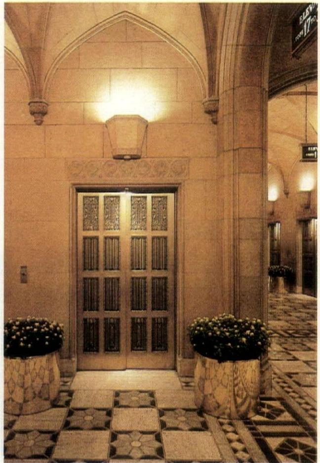
The Gothic ornamentation of the entry arch is illuminated by 90-watt halogen lamps, which are used as uplights behind the sconces. Cored into the bottom side of the wall sconces, 50-watt MR 16 recessed damp label fixtures are recessed and angled slightly inwards to create an asymmetric effect in each niche. One more 500-watt high-bay quartz downlight was added in the center of the entry's compound arched ceiling to brighten the floor and threshold.
