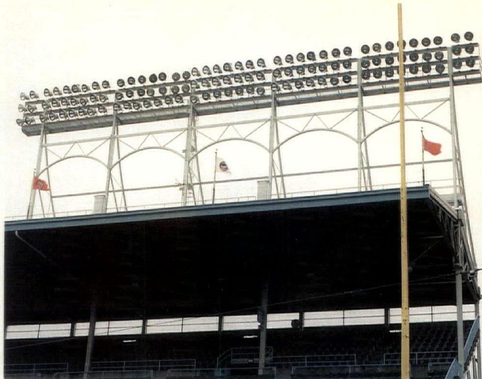
eliminate occasional head-on viewing of floodlights, but this should be casual viewing and not required during the playing or viewing of a sport. Floodlights must therefore be located out of the direct line of sight of any play. They must be mounted high above the normal viewing angle of players and spectators. Install floodlights where players are least likely to look, which varies with the sport being played.
