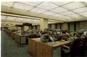
**MULTIFUNCTIONAL LIGHTING:** An indirect, fluorescent system provides illumination for cross-floor communication, and minimizes glare on computer screens.
