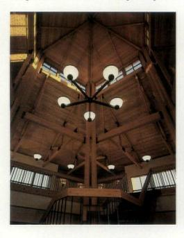
WEST BEND GENERAL CLINIC: The consistent styling of the fixtures from the circular atrium to the perimeter corridors is provided by variations on the theme of extruded aluminum arm stocks supporting luminous acrylic diffusers that each house a 175-watt metal halide lamp. Photo courtesy of Visa Lighting.
