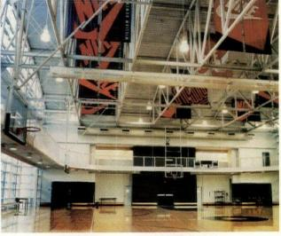
GYMNASIUM: Metal halide luminaires equipped with prismatic glass reflectors are suspended from the domed ceiling to provide 70 footcandles average maintained on the gym floor.
