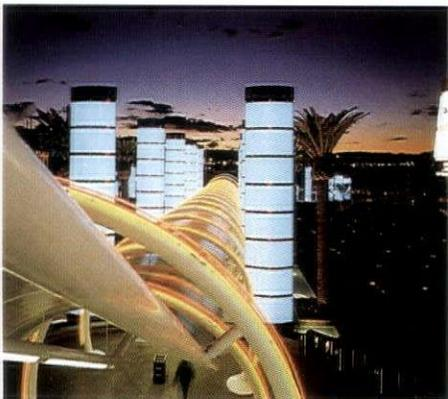
Ranging in height from 18-38 ft., the glowing pylons flank a neon-lit, spiral walkway that leads to the casino. Constructed of perforated metal backed by an opal acrylic sheet, the pylons house 15mm neon tubes running top to bottom, spaced 6 in. apart, divided by a deeper reveal housing MR11 spots fitted with red lenses. The tubes are red,
