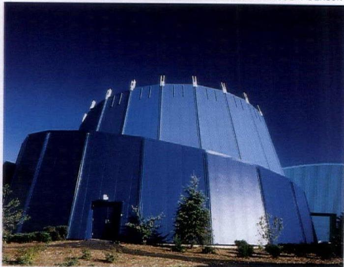
CONCEALING THE EIGHT SOURCES FROM VIEW ACHIEVES THE DRAMATIC EFFECT OF THE ENTRY PAVILION: POLE-MOUNTED METAL HALIDE FLOODLIGHTS ARE AIMED AT BOTH SLOPES OF THE ROOF (THE LAMPING IS CONSISTENT BUT THE DISTRIBUTION AND ANGLE OF THE FIXTURE VARIES) AND DOWNLIGHTS ARE MOUNTED TO THE INNER AND OUTER PERIMETERS.
