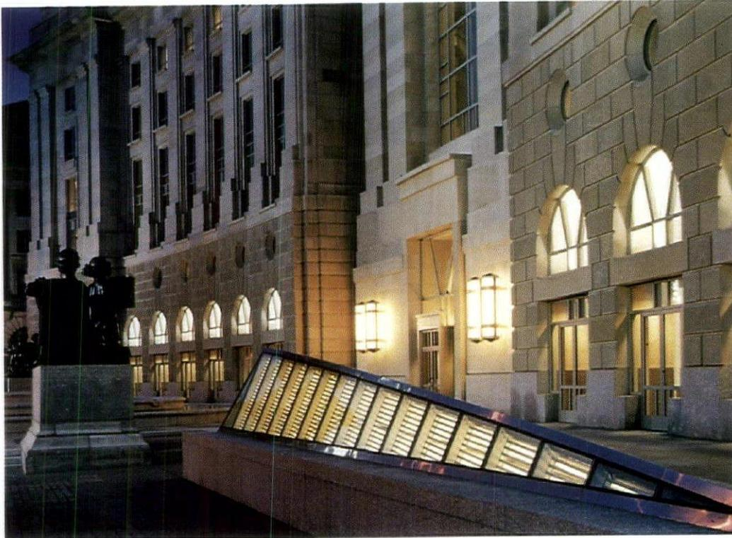
LEFT: OUTSIDE THE RONALD REAGAN BUILDING, A CRESCENT-SHAPED SKYLIGHT WITH A SUN-SCREEN MADE OF METAL TUBES SPACED 1 IN. ON CENTER INTIMATES THE MODERN GEOMETRIC FORMS THAT CHARACTERIZE THE INTERIOR. THE SUNSCREENS ARE UPLIGHTED WITH CUSTOM WALL-BRACKET-MOUNTED FLUORESCENT FIXTURES, WHICH PROVIDE AMBIENT LIGHT FOR THE CAFETERIA BELOW. DUAL SCONCES MADE OF STAINLESS STEEL AND GLASS AND FITTED WITH FLUORESCENT LAMPS MARK THE MAIN ENTRANCE AND COMPLEMENT THE NEO-CLASSICAL-STYLE ARCHITECTURE.
