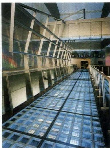
THIS HIGHLY ARTICULATED, THOUGH SEEMINGLY WEIGHTLESS, METAL BRIDGE, SUSPENDED THROUGH THE HIGH-VOLUME ATRIUM, IS FLOORED WITH GLASS BLOCK TO ALLOW LIGHT TO TRANSMIT INTO THE SPACE BELOW, ADDING TO THE EXCITEMENT OF THE SPACE.
