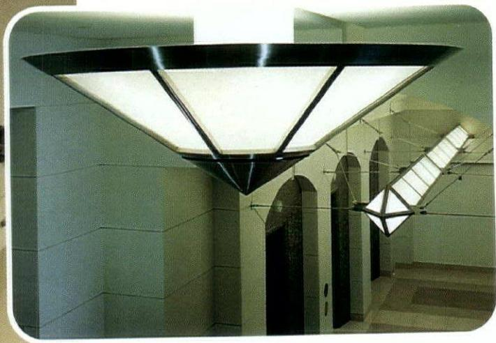
LEFT: ANOTHER EXAMPLE OF THE VARIOUS GEOMETRIC SHAPES THAT ARE CRUCIAL TO THE LIGHTING DESIGN OF THIS PROJECT. SUSPENDED BY STAINLESS-STEEL RODS IN AN ELEVATOR BAY, A 22-FT.-LONG LINEAR FIXTURE IS ILLUMINATED WITH F40T8 AND F32T8 FLUORESCENTS. INSET: A SERIES OF CUSTOM-DESIGNED CONED-SHAPED CHANDELIERS, EACH CONTAINING TWELVE 39W T5 TWIN-TUBE COMPACT FLUORESCENT LAMPS, MARKS THE DECISION-MAKING POINTS ALONG CIRCULATION ROUTES.
