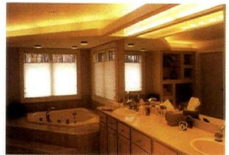
**FIGURE 5**—A DROPPED SOFFIT OVER THE LAVATORY/VANITY AREAS IN THIS MASTER BATH USES BOTH INCANDESCENT AND T8 FLUORESCENT STRIPS TO PROVIDE A DIRECT/INDIRECT DISTRIBUTION. THIS CUSTOM FIXTURE PROVIDES BOTH TASK AND AMBIENT LIGHTING. PHOTO ©ROBERT J. EOVALDI
