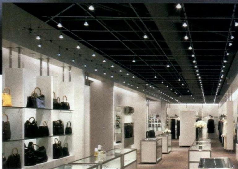
**V/A**, one of nine systems from Bruck, is a low profile track system that can easily change directions and elevations. Available in straight or curved segments, in chrome, matte chrome, or gold finish.
