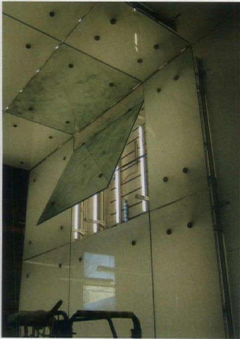
A full-scale mock-up (left) was constructed to test the placement of the lighting—linear fluorescents and RGB LED strips—used to backlight the laminated glass panels of the lobby's walls and ceiling. As seen in the section details below, careful attention was paid to the assembly of lights sources, glass, and art film to create an even but nuanced illumination.
