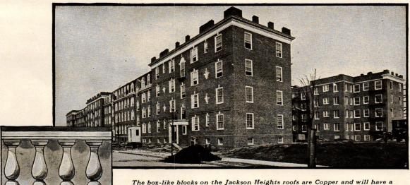
The box-like blocks on the Jackson Heights roofs are Copper and will have a Copper balustrade joining them as shown in the small sketch. 16 to 24 ounce Copper is being used.
