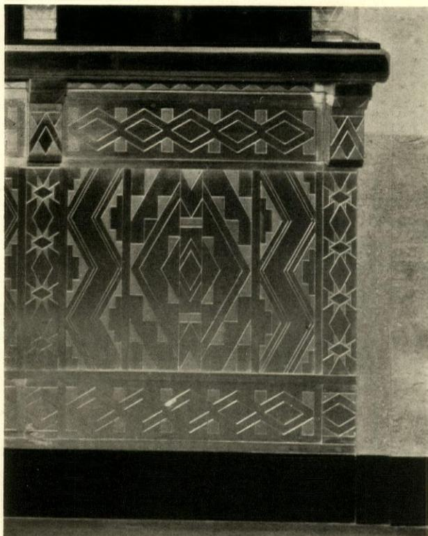
*A detail of a bank counter base produced chiefly by the routing machine shown below*
