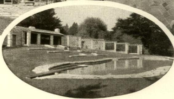
CONCRETE, in many forms, has been skillfully employed by the architect in designing this home. The exterior walls are of concrete masonry units, in slightly irregular sizes and varied colors. Building frame and floors throughout are of reinforced concrete—*one unit*, of utmost strength and rigidity. The roof is attractively tiled. So constructed, a home is *firesafe* and long enduring.
