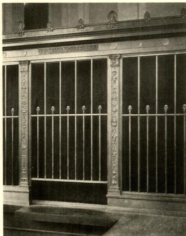
*A typical banking counter-screen, such as is being produced more and more frequently in extruded metal embellished by cast work*
