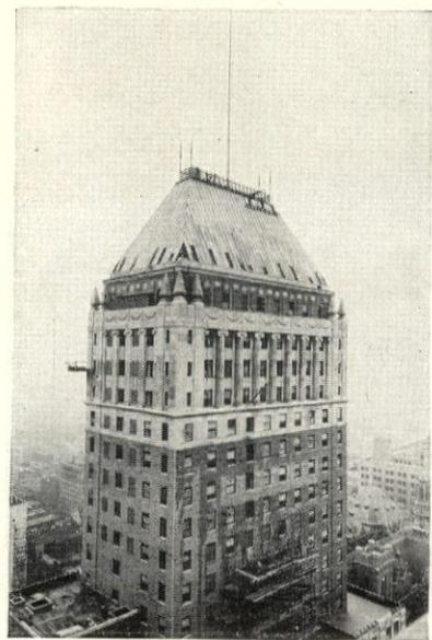
Tower portion of Newark & Essex Bank Building. ALBERENE STONE SPANDRELS used at 32nd and 33rd floor levels—on all four elevations.
