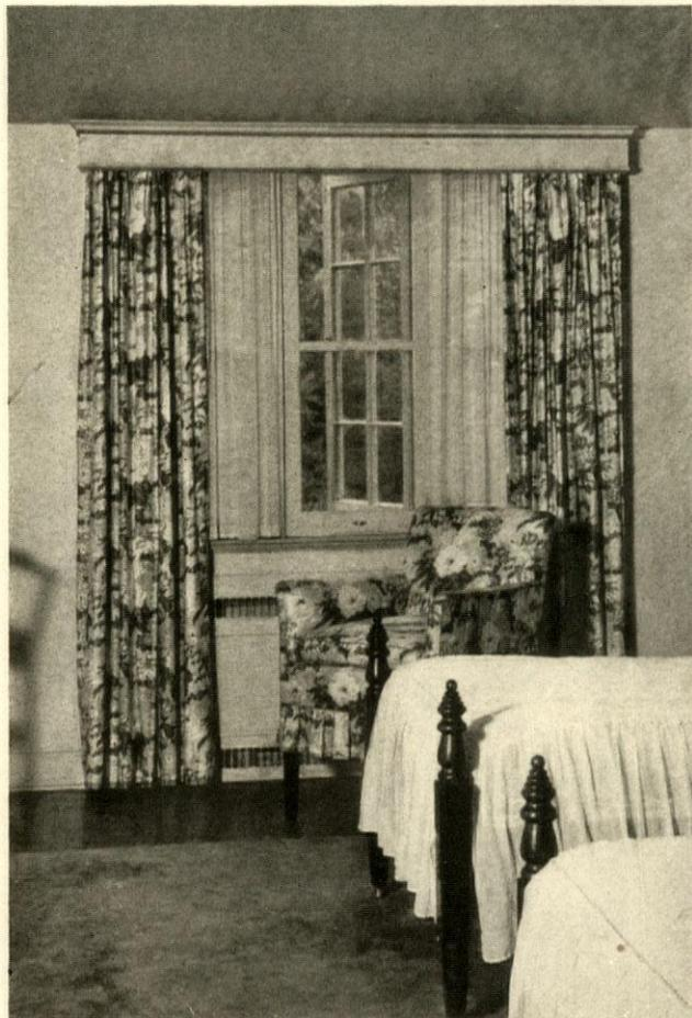
*Wood casements, with wood frame screens inside, and boxed head for draperies. Ethel A. Reeve, Inc.*
