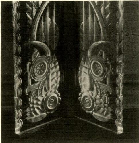
*Detail of a console table in "carved" (sandblasting through stencils) glass lighted from the inside edge, designed and executed by Feybusch Associates, New York*
