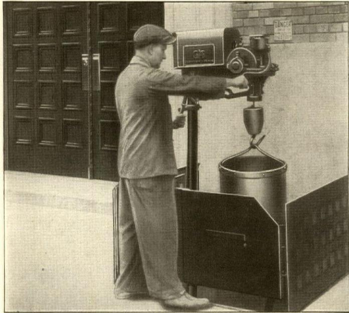
*Model E Electric Hoist as used in bank buildings.
