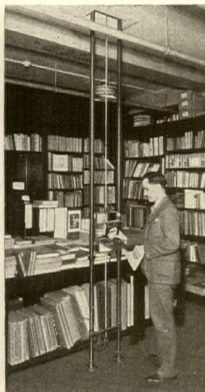
Main floor view of Sedgwick Lift used for handling books between main floor and the mezzanine. Various styles of carrier available to meet specific needs.
