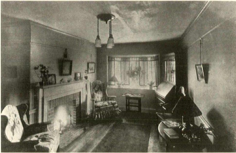
*Here is one of the living-rooms in which Mr. Ham has used wall board without plaster. He runs his lengths horizontally, covering the joints with a cornice moulding, a low picture moulding, a chair rail, and the baseboard. The greatest difficulty, of course, is a vertical junction at a projecting angle, which he solves with a special corner moulding*
