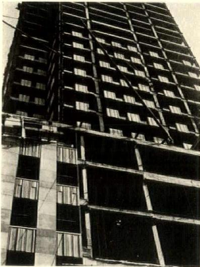
*Limestone following the cast aluminum spandrels up the steel frame. Rockefeller Centre, New York City*
