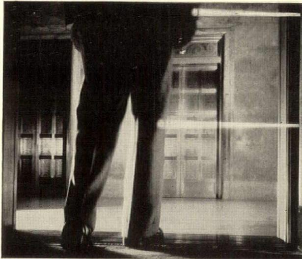
Westinghouse Safe-T-Ray. Now swift-moving, power-operated elevator doors are provided with rays which do not allow the doors to close if any one is stepping in or out of the elevator—a much needed safety feature.
