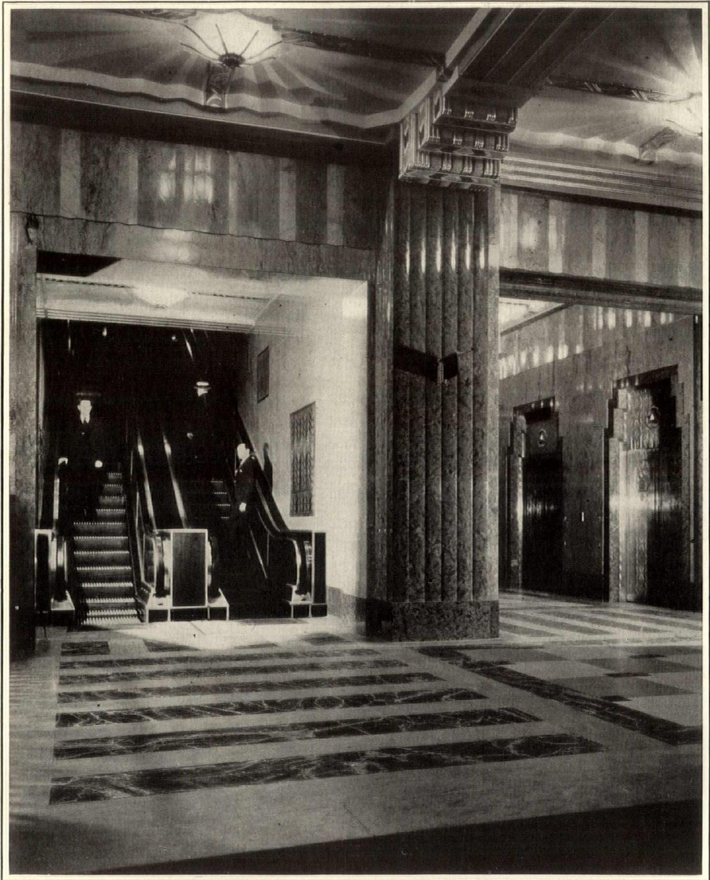
**WE WISH** to direct your attention to this photograph because it illustrates an important building trend of today, namely, the use of escalators to supplement elevators. These escalators handle the heavy traffic of lower floors and leave the elevators free to serve upper-floor tenants. Photograph of the new Cities Service Building, of New York City. Sixty Wall Tower. Escalator and elevator installation by Otis Elevator Company.
