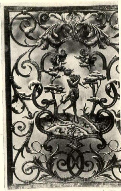
*The traditional wrought-iron grille formed of straight bars is given a new interpretation by rhythmic spacing, with intersections overlaid by leaves and tendrils, in this vestibule door below, in the residence of F. G. Achelis, Greenwich, Conn. H. T. Lindeberg, architect; executed by The Iron-Craftsmen*
