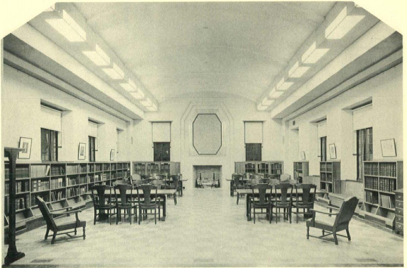
*Reading-room at night. Built-in lighting in the ceiling is an innovation proposed by the architects which has proved to be very successful. It eliminates both lights on the tables with their resultant eye strain and clumsy and inefficient chandeliers. Neighbors leave their homes in the evening to come and read in the library on account of the good light*
