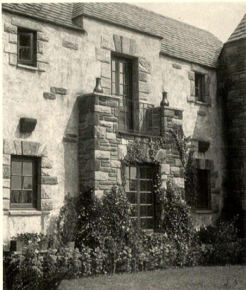
*The deeply embrasured window on the southeast side of the living-room, with a balcony above. Copings and sills throughout the house, as well as the paving, are of flagstone. The roof is of black slate*
