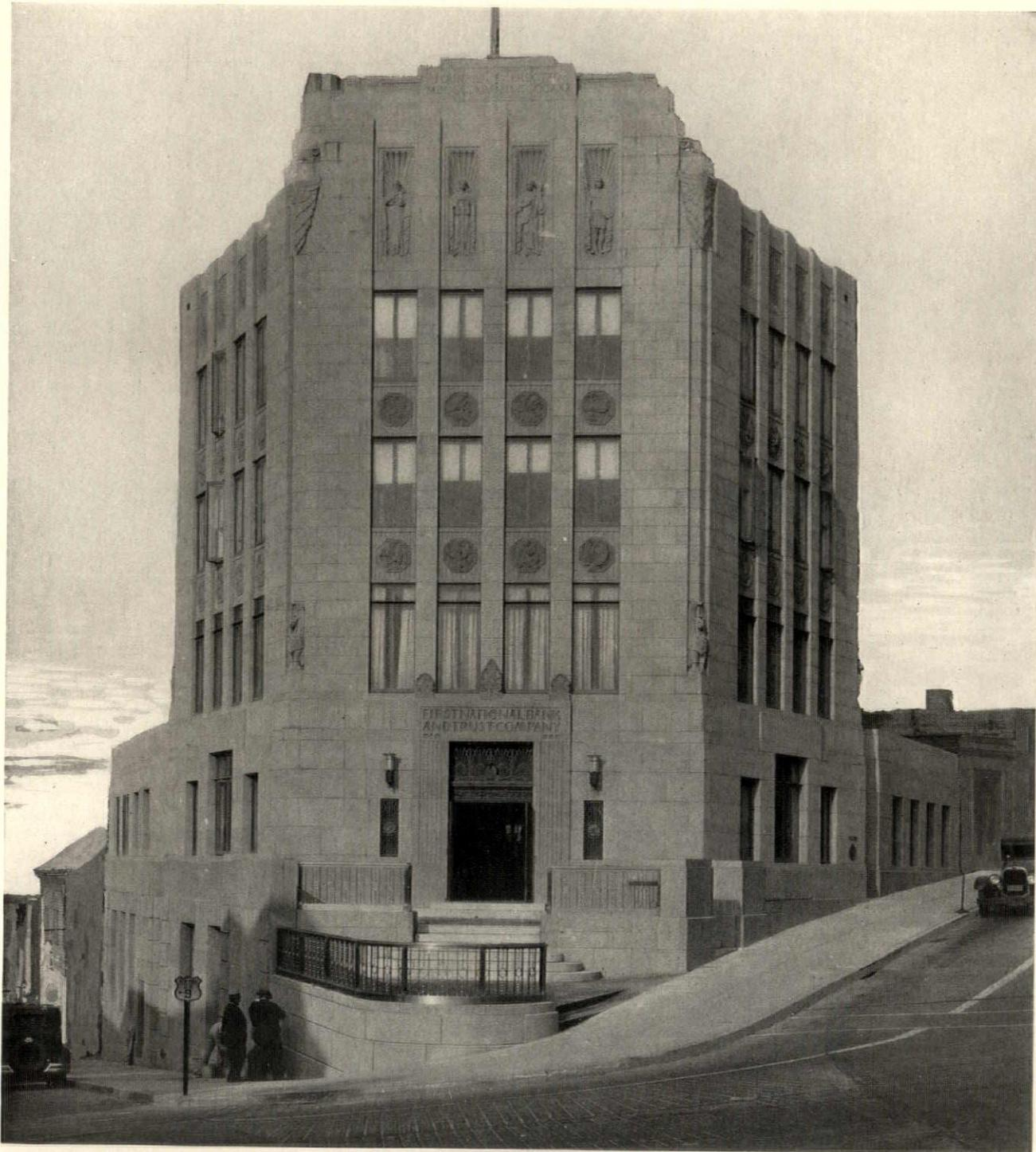
*The triangular corner plot for bank use is not uncommon, but when combined with a steeply shifting grade as shown here, it presents some difficulties to the architect. The building is of fire-proof construction, the exterior walls above grade being faced with cast stone resembling granite. Doors and grilles are of bronze, the windows of steel*
