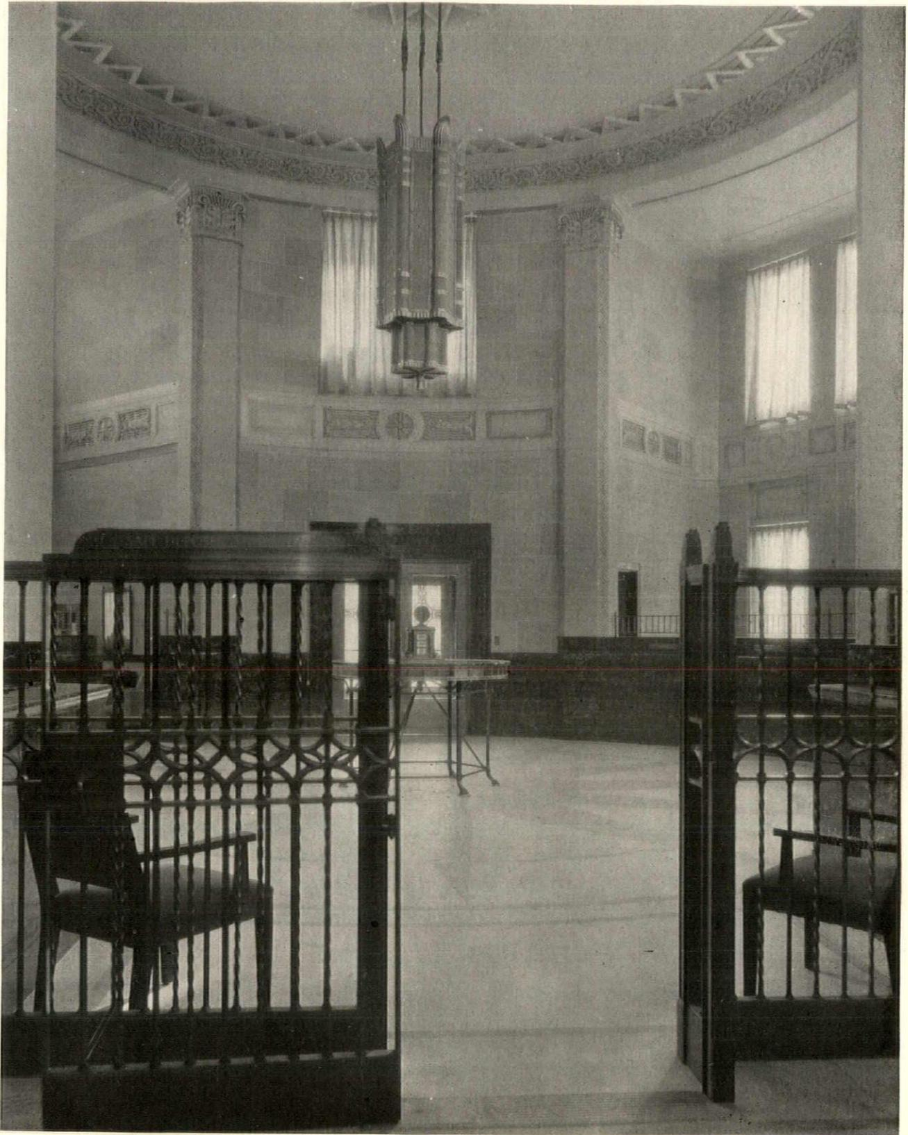
*As finally developed, the hexagonal form of the banking-room is cut by the entrance segment, without, however, detracting unduly from the original scheme. The ceiling here is twenty-three feet high, lighted and ventilated on all six wall surfaces by windows in the upper portion leading directly to the outside air and light. The general color scheme of the room is that of Caen stone with decorations in old ivory*
