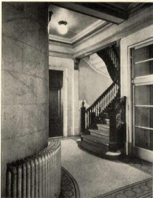
*Inside the Cities Service Company's building, R. M. Karger, architect, has done away with the old radiator, has installed modern lighting, replaced the old floor with terrazzo, and redesigned the elevator entrances*
