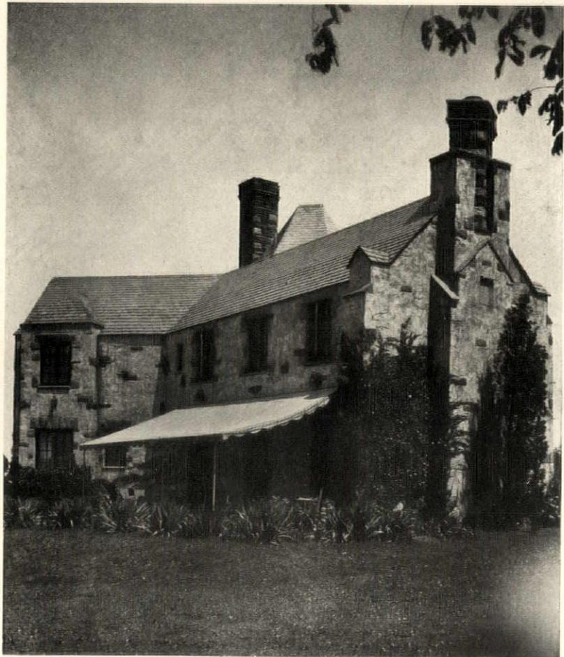
*The terrace side, which commands the extensive view over the Whitemarsh Valley. The angularity of the plan resulted not only from the purpose of securing the best views for the principal rooms, but also because of the sharply sloping site*
