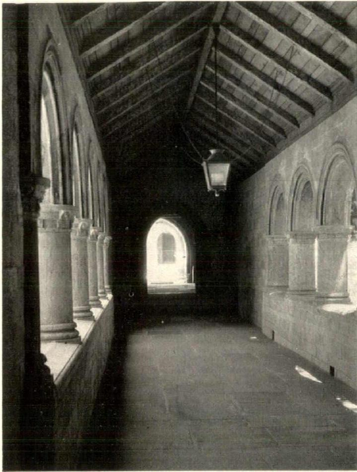
*Looking through the arcade built on top of the dam. For the structure the architects have used concrete blocks with cast stone*
