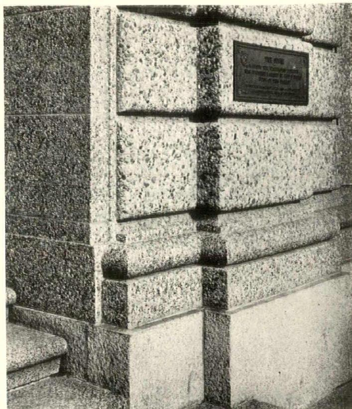
*The first structure built with architectural concrete made by the new technique—a technique in which the surface aggregate is predetermined and prearranged*
