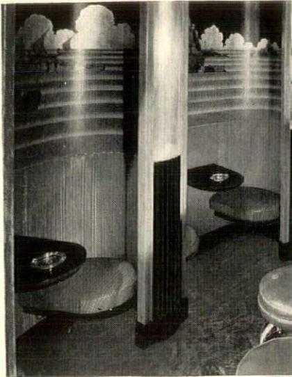
*St. Clair Hotel, 160 E. Ohio St., Chicago, Ill. Oman & Lilienthal, Architects. Murals by Alexander Rindskopf. Circular bar 8' in diameter. Workboard of Stainless Steel, including drainboards, waste chutes, storage racks, etc. The beer is mechanically refrigerated, having an under-counter Brunswick Instantaneous Beer Cooler. Upper Left: Note clever, compact, efficient arrangement of seats and table with the booth — allowing sufficient room for 2 guests.*
