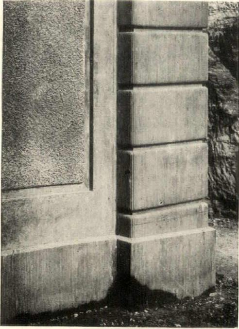
*On the left, a structural concrete wall in which there is no provision for color other than that of the natural cement*
