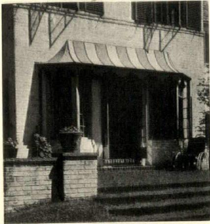
Woodmere, Long Island. The roof of the hood is of copper with standing seams, the spaces between these seams being painted alternately dark blue and China yellow. The copper valance, which is backed up with thin wood, is also painted.
