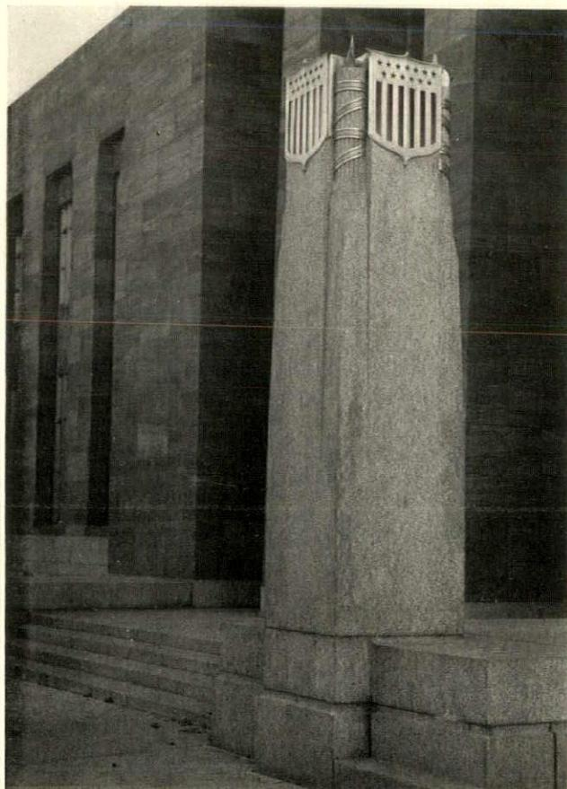
*Principal corners were reduced by entasis to provide a base for the sculpture. All exterior angles are slightly rounded, increasing the radius toward the top*
