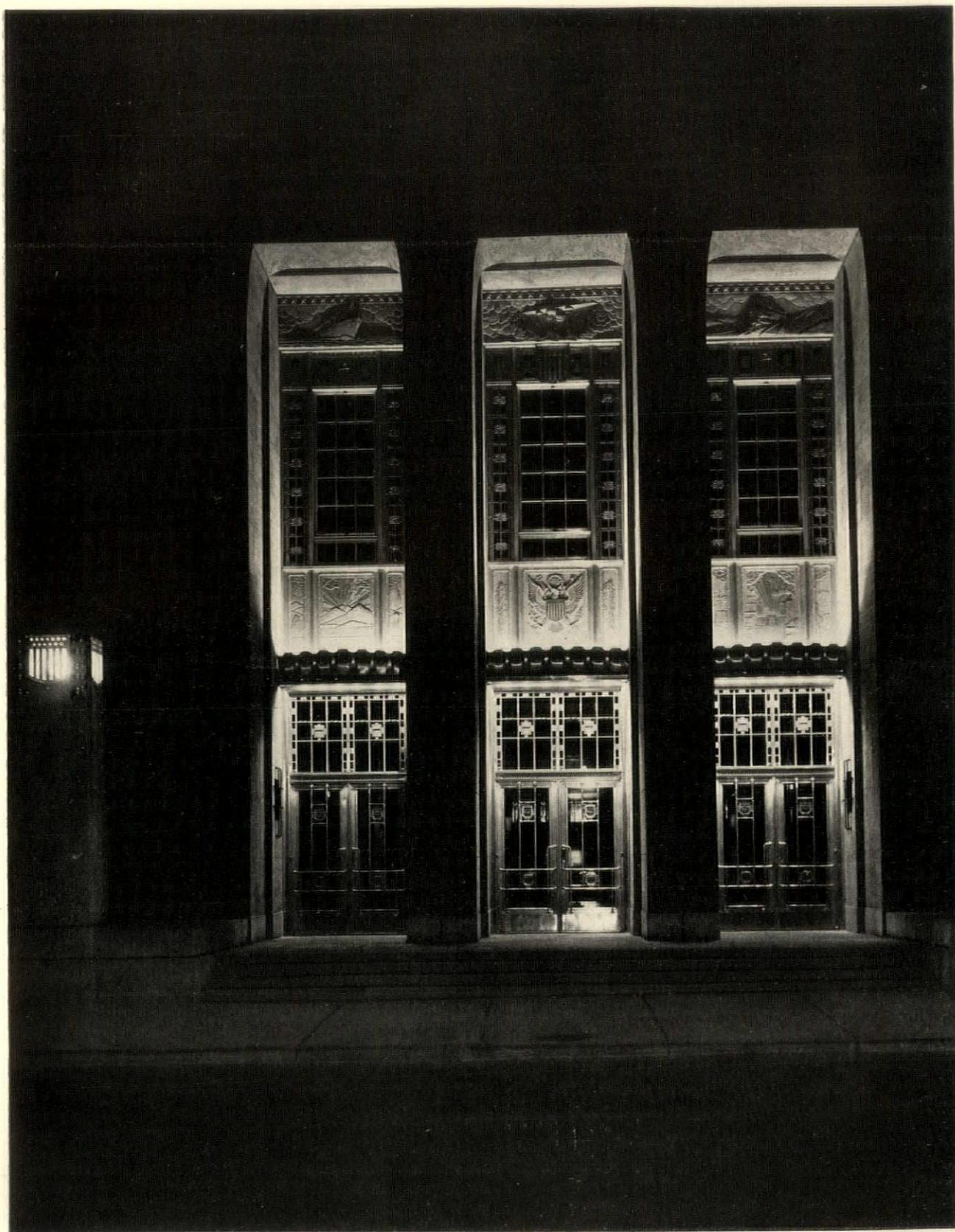
*Main entrance at night. Windows, doors, and other exterior metal features are of satin-finished aluminum. Spandrels and other cast work have a dust-blast background with ornament high-lighted*
