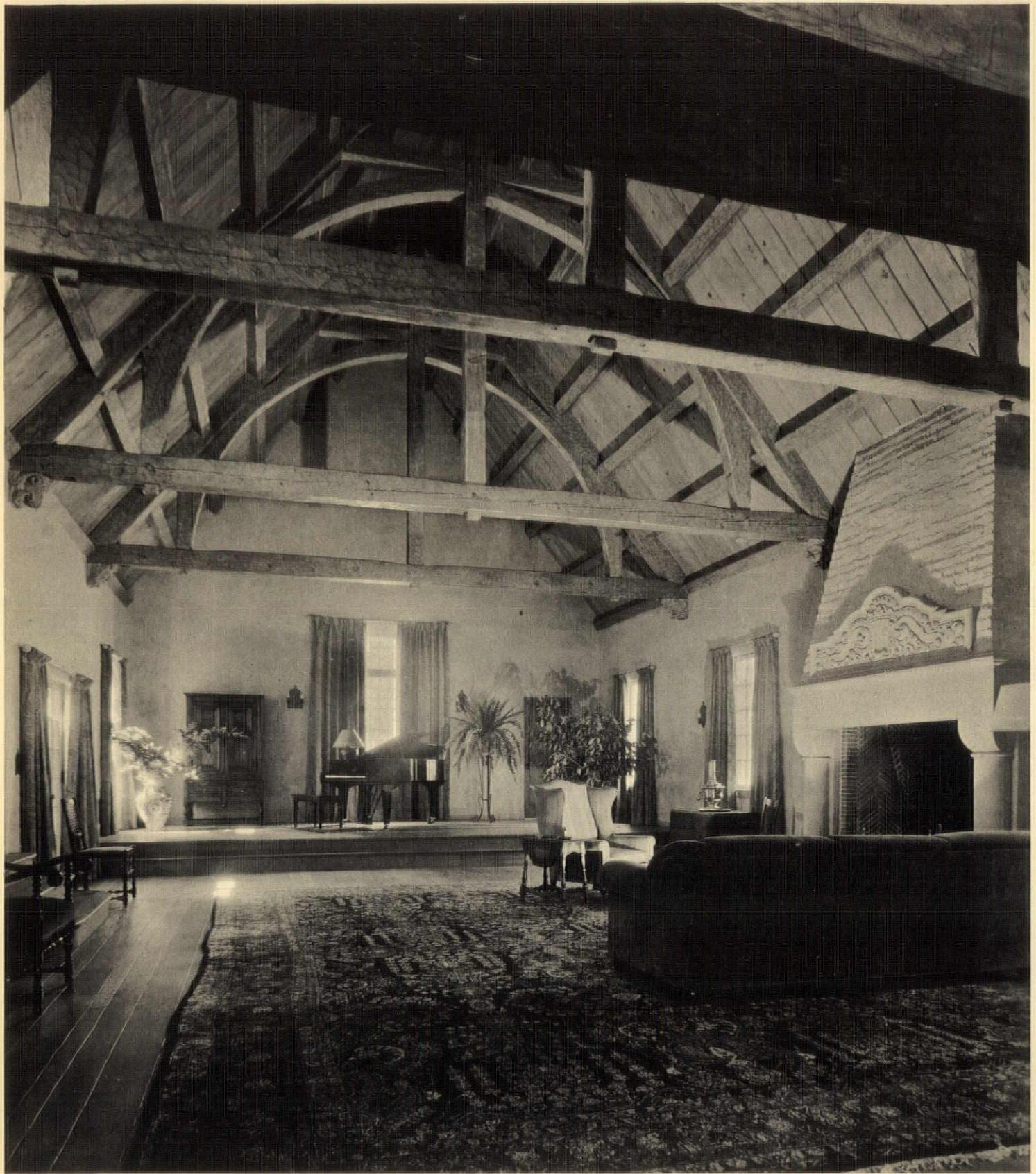
*An acoustical plaster was used for the walls, with which a large amount of mineral wool was incorporated. The color, too, a dull straw, was mixed with the plaster*
