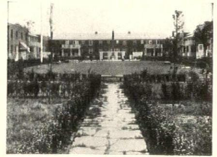
Fig. 26. At left, a view through the middle portion of a block developed in the customary manner utilizing the rear yards and garages on an alley. Contrast with this (at right) the center yard court of a Sunnyside block, in which the distance of houses from rear to rear is the same as in the alley scheme. Garages are assembled elsewhere in groups
