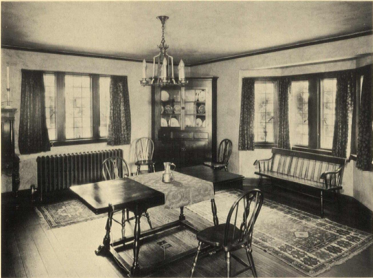
*The dining-room has the same oak plank floor as the living-room, scraped across the grain and finished dark brown. Here the plaster has a texture slightly rougher than a float finish. The trim here, as throughout the first floor, is of oak with a dark brown stain*
