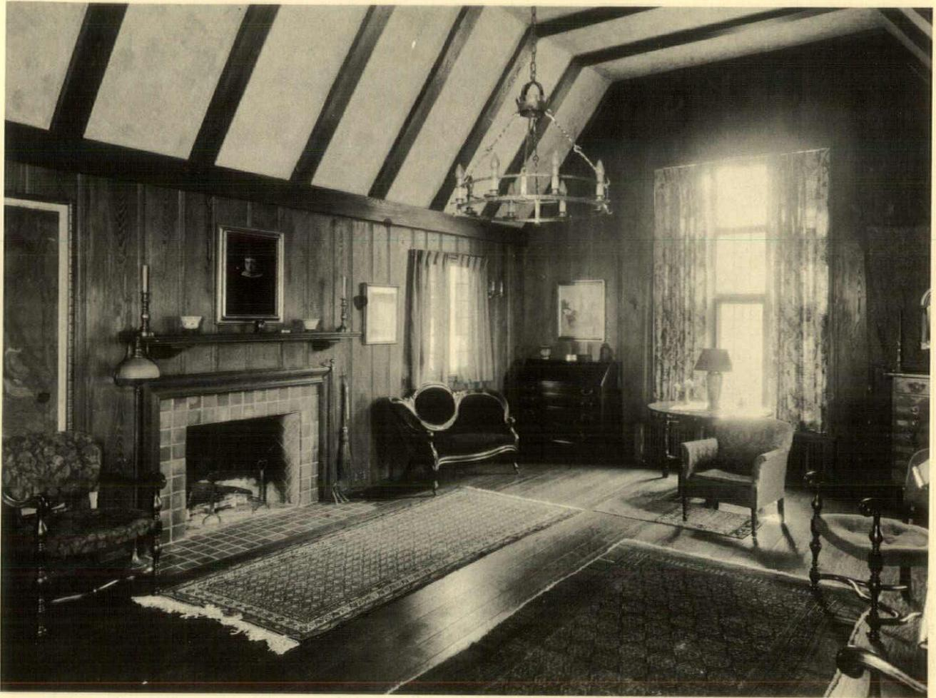
The feature of the interior is a two-story living-room with its adjoining book alcove, both of which are faced with vertical chestnut boards, burned with a torch and waxed. Floors are of plank in random widths, showing the wooden pegs. It has been scraped across the grain, and finished in a rich brown. The tiles for the fireplace facing are a dull reddish brown. Between the ceiling beams the plaster is of a cream tone, slightly antiqued
