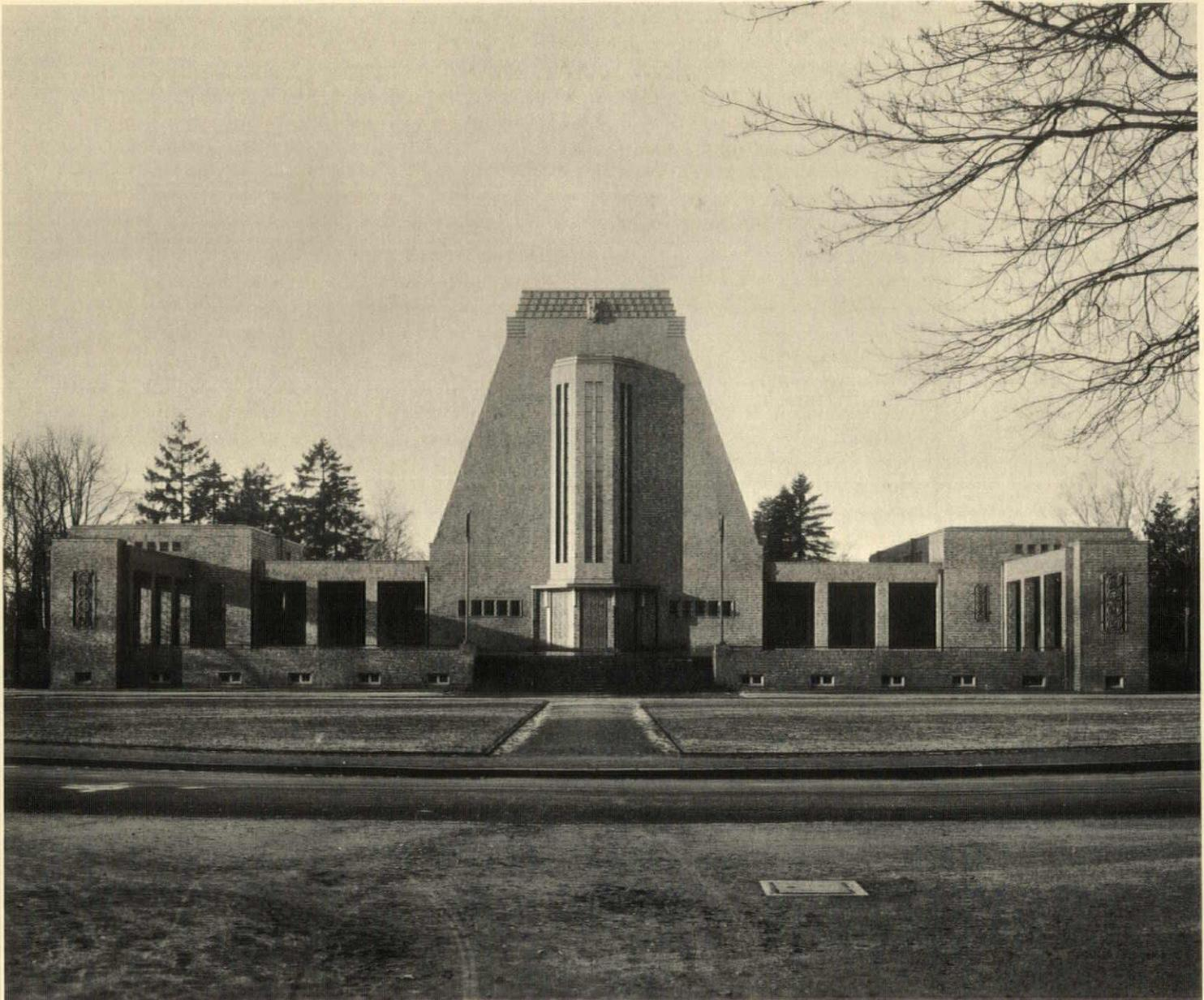
*The structure is of reinforced concrete faced with brick of a blue-red color. All of the ornamentation—which is very much restricted—is in brick. There is a broad terrace across the front with the entrances through the loggia*
