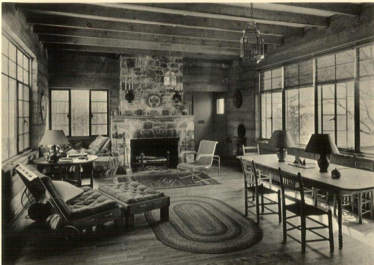
*In the living-room the reinforced-concrete walls, laid up with movable molds, were left untreated. Ceiling joists were stained, and they have insulating board between them under the second floor. The fireplace is of the type which also heats two supplementary ducts of air*
