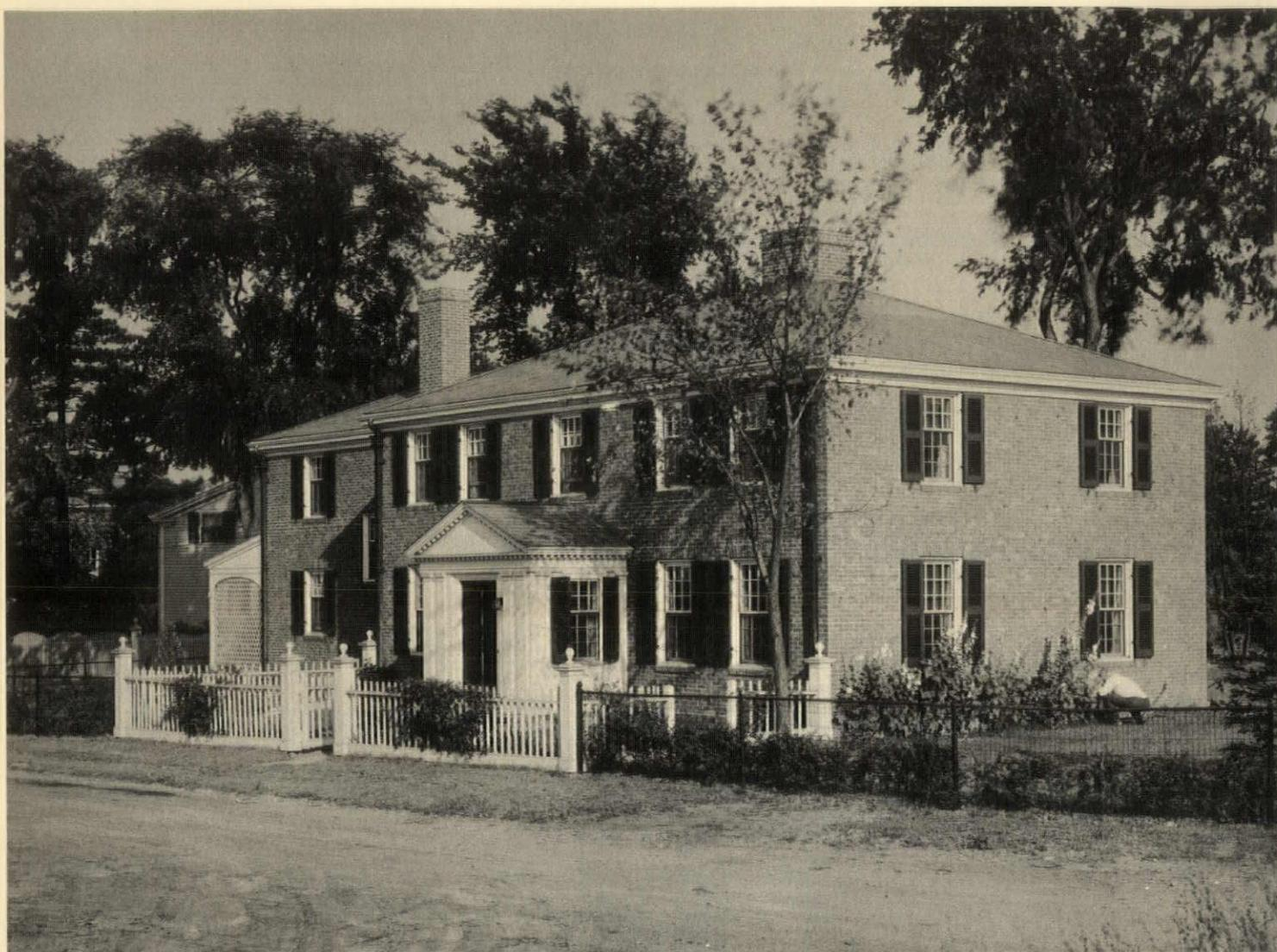
*The house is of brick veneer on a wooden frame, the brick used being a common water-struck New England brick laid with a wiped joint of light gray mortar. The trim is wood painted white, with the exception of the blinds and front door, which are dark green. A sea green Vermont slate is used for the roof*
