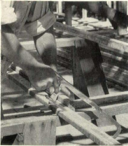
*The structural members are prefabricated to finish size, but may be cut with a hacksaw*
