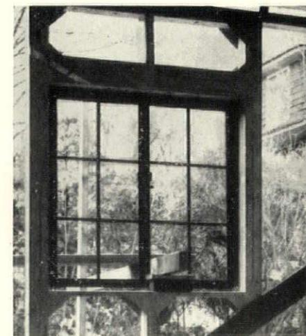
*A steel window in its buck. Note that this is secured to studs and plate by 22-gauge gussets*
