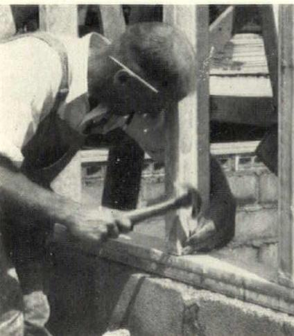
*Studs are toe-nailed to sill, and because of their metal sheathing they cannot split as wood studs frequently do*
