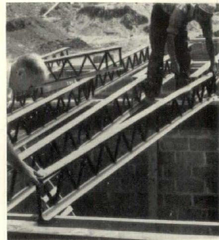
*Spacing the floor joists, in the top and bottom crimped web of which is a fireproof core to receive nailing*
