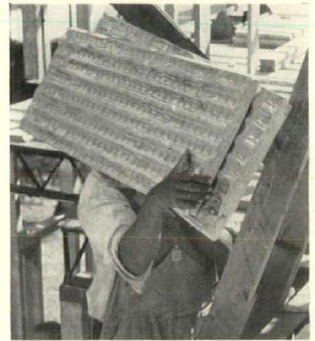
*Ship-lap floor slabs,  $15\frac{1}{2}$ " by 4', reinforced by Ecod fabric and stud bars, are light enough for easy handling*
