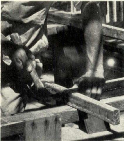
*The carpenter nails together a door or window buck just as he is accustomed to do in wood construction*
