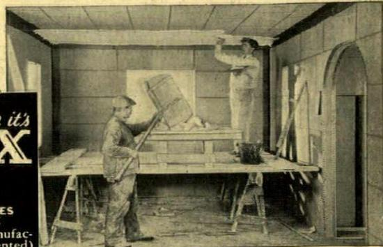
*Celotex as Plaster Base builds as it insulates*
