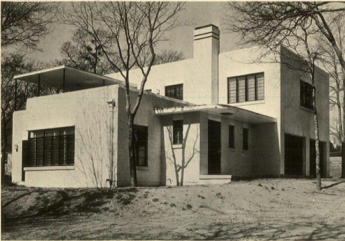
Steel casement windows are used throughout, and the concrete tile has been given a coat of cement paint
