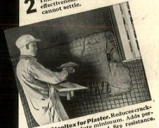
**3** **J-M Steeltex for Plaster.** Reduces cracking to an absolute minimum. Adds permanence, strength and fire resistance.
