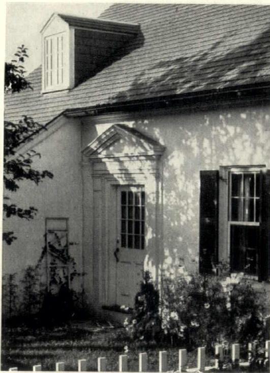
*white, and the green blinds and white picket fence echo the New England tradition. Inside, the block walls are furred with fiber board with the joints smoothed to afford directly a surface for wall-paper. There is a basement under the house, and its total cost was \$6000*
