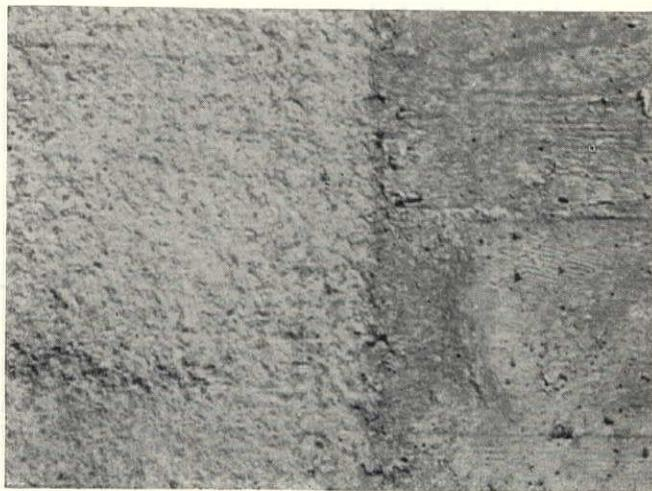
FIG. 3.—SURFACE OF "PICKED" CONCRETE.
