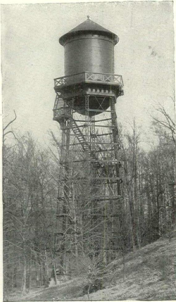
**W**E make a specialty of the design and construction of steel tanks for fire protection and general service. Our elevated tanks give a positive direct supply of water under pressure which is independent of the operation of any machinery to maintain the pressure until the tank is entirely empty.
