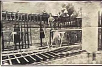
*Brown Apartment Building, Indianapolis, Ind. C. A. Wallingford, Architect. Arthur Sanford, Contractor. Construction view showing Metal Lumber Joists and Studs of floor and partition construction.*
