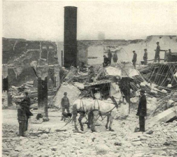
REMOVING DEBRIS TO CHUTE WITH TEAM AND SLIP SCRAPER
