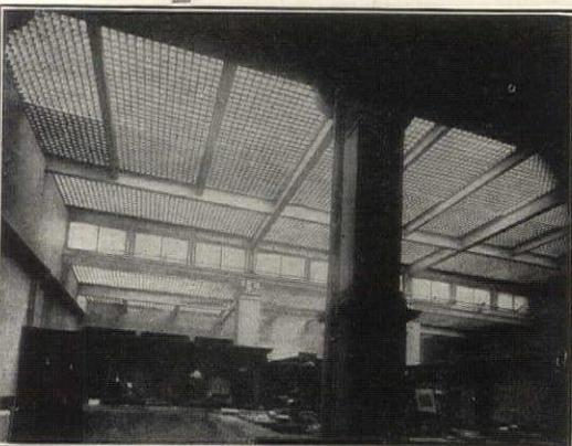
Banking room under Court. Raydiant makes artificial light unnecessary.
