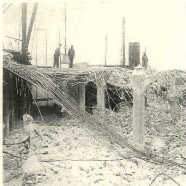
WRECKING FLOOR SLABS WITH BALL
