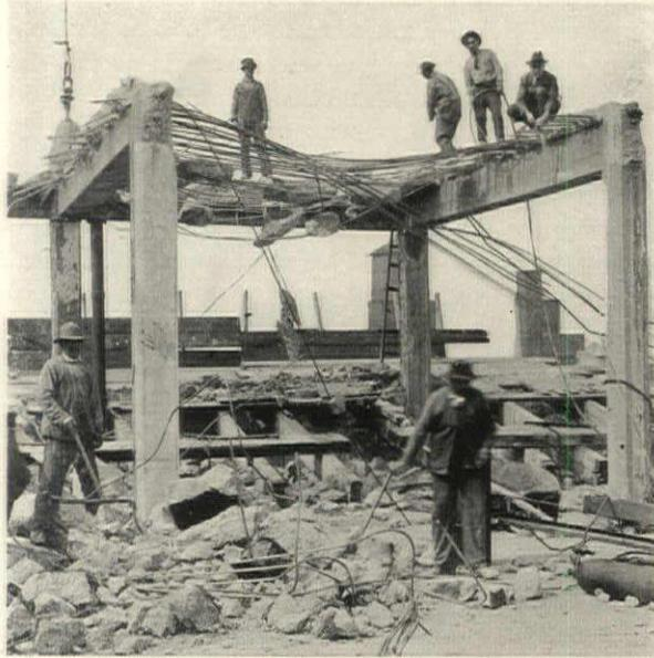
CUTTING SLAB BARS WITH ACETYLENE TORCH
