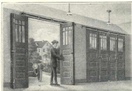
Interior view double entrance garage, both doorways equipped with 4-door Slidetite hardware.
