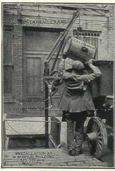
Model B is designed primarily for use in buildings where it is possible for wagons to drive up alongside of hatch. It eliminates the necessity of rehandling at the sidewalk—a saving in both time and labor.
