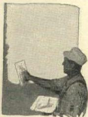
These results are due to the purity and peculiar natural composition, plus the chemical content of the limestone rock from which Ohio White Finishing Lime is made. Its "fatness" or plasticity makes it spread easily and enables the plasterer to obtain maximum coverage with minimum effort.
