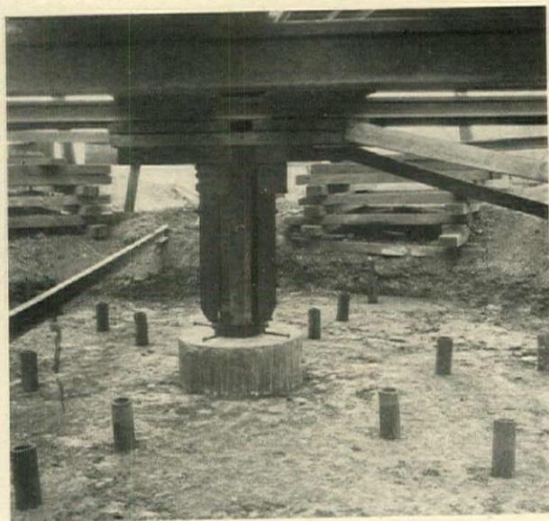
SHOWING THE BASE OF THE LOADED MAST RESTING ON THE TEST BLOCK AND BOLTS PROTECTED BY TILES
