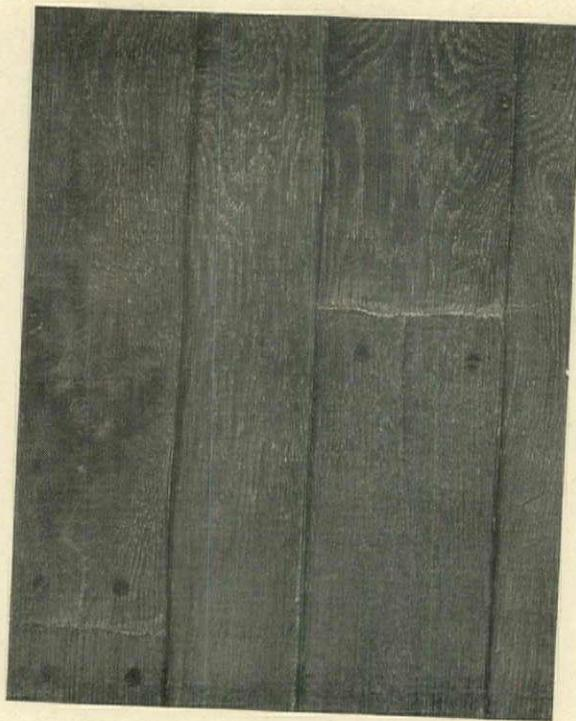
Section of oak plank flooring typical of Jacobean rooms. The planks are of random widths, rough hewn, and the effect is crude and free-hand, but in keeping with the spirit of the period
