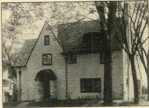
Chicago common brick finished with Cabot's Old Virginia White; roof stained with Cabot's Shingle Stain.
