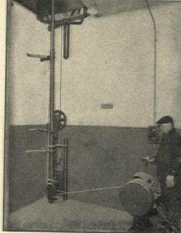
*Model D Electric G&G Telescopic Hoist at Mergenthaler Linotype Co., Brooklyn, N. Y. Test showed 78 cans of ashes raised and lowered in 1 k.w.h.*
