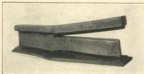
Slitting rolls separate Head and Flange from Web as rail comes from the heating furnace.
