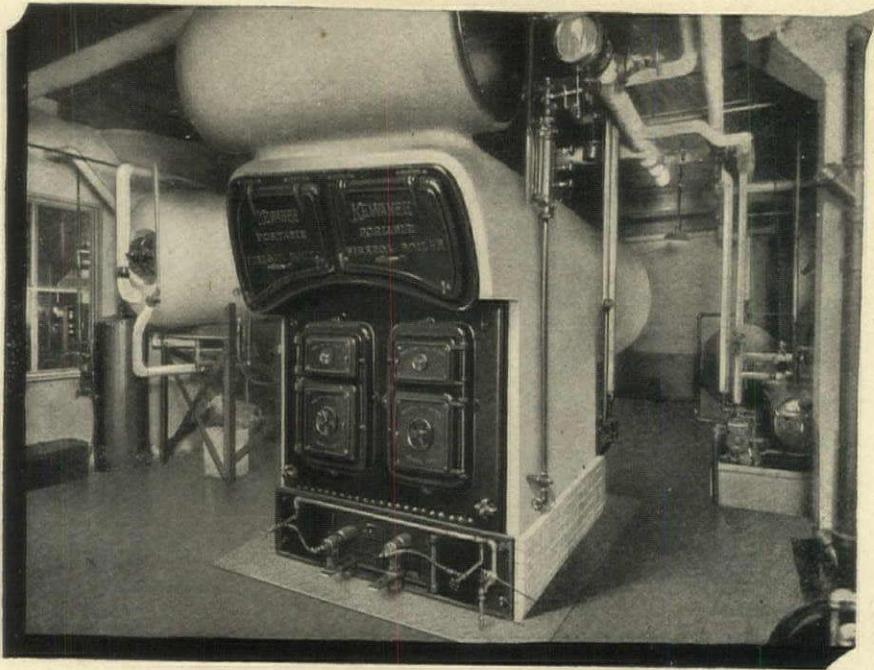
Time is an element entering into the economy of oil flame formation. The high and wide mixing space in Kewanee boiler fireboxes provides an ideal chamber in which combustion is perfected so that the flames do not impinge on the tube surfaces.
