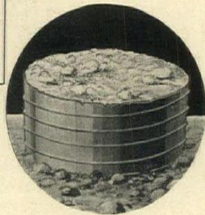
Raymond Concrete Piles are poured today exactly as they were 21 years ago — time has simply confirmed the wisdom of pouring each pile into a spirally reinforced steel shell and leaving the shell in the ground.
