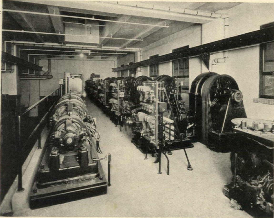
VIEW OF ELEVATOR MACHINE ROOM IN DEPARTMENT STORE FOR JOSEPH HORNE COMPANY, PITTSBURGH, PA., SHOWING THE APPARATUS REQUIRED FOR VARIABLE VOLTAGE CONTROL. AT THE LEFT ARE THREE MOTOR GENERATOR SETS; AT THE RIGHT THE CONTROL PANELS AND WINDING MACHINES
