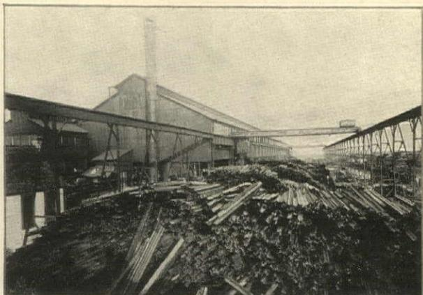
Thousands of tons of Rails awaiting their turn to be reborn to new usefulness through the heating furnace and mill.
