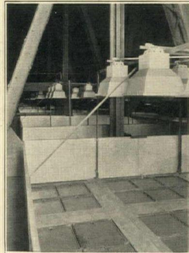
One battery of these reflectors is over each of the 40 ceiling panels. The metal curbing around the panel is to retain the light and to afford a background when the ceiling is viewed from an angle. Such care and forethought is typical of all Frink installations.
