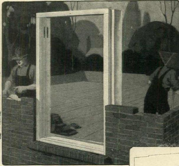
The double shoulder on the sill makes the Andersen Box Window Frame water- and wind-proof.
