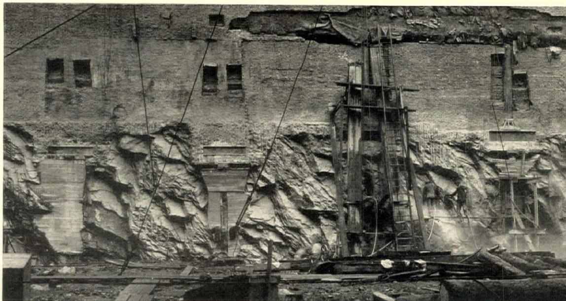
VIEW OF WEST WALL OF PRESENT BUILDING, SHOWING STEEL STRUT AND CONCRETE UNDERPINNING OF EXISTING FOUNDATIONS. HEAVY TIMBER SHORES USED TO PREVENT LATERAL MOVEMENT OF THE EXISTING COLUMNS
