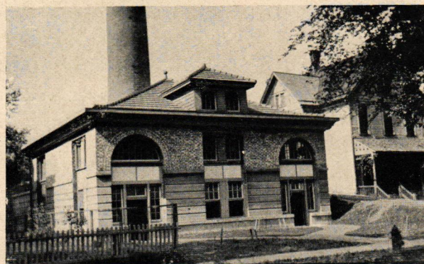
REFUSE INCINERATOR AT OAK PARK, ILL.
