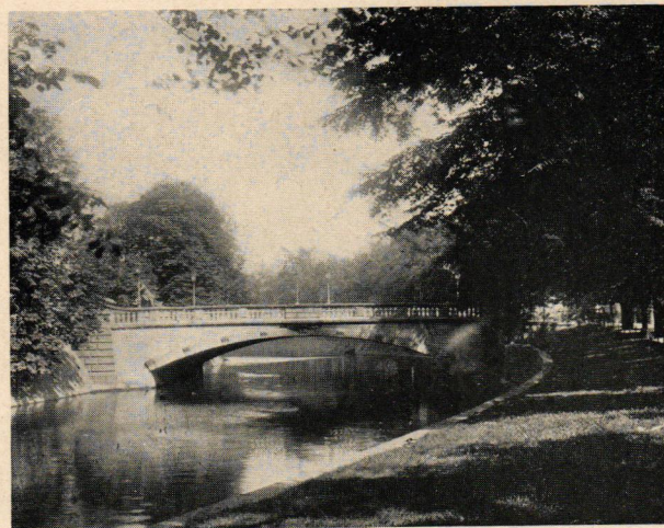
BRIDGE OVER CANAL, MAGDEBURGER STRASSE, BERLIN
