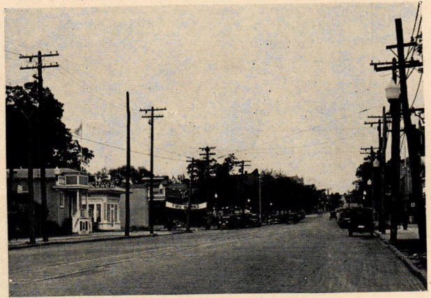
FIG. 2. MAMARONECK, N. Y., HAS INSTALLED NOVALUX BRACKET ORNAMENTAL FIXTURES ON THE WOOD TROLLEY POLES. THE EFFECT IS QUITE PLEASING
