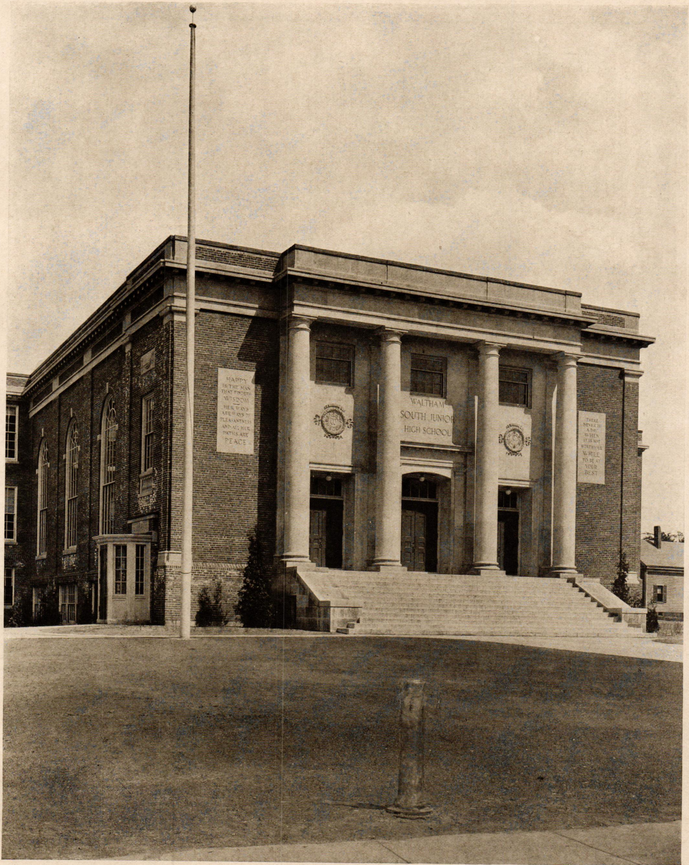
SOUTH JUNIOR HIGH SCHOOL, WALTHAM, MASS. A COMBINED SCHOOL AND COMMUNITY BUILDING KILHAM, HOPKINS & GREELEY, ARCHITECTS
