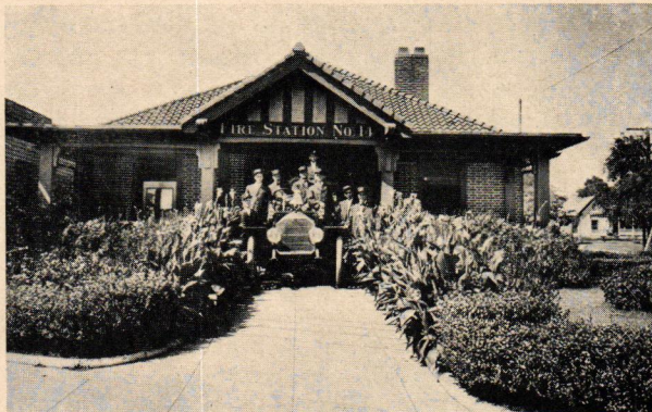
A BUNGALOW TYPE OF FIRE ENGINE HOUSE WHICH CONFORMS WITH THE SURROUNDING IMPROVEMENTS
