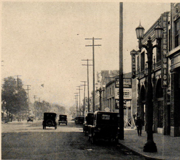
FIG. 5. HOLLYWOOD, CAL., USES AN ORNAMENTAL POLE ON WHICH ARE MOUNTED TWO ORNAMENTAL LANTERNS
