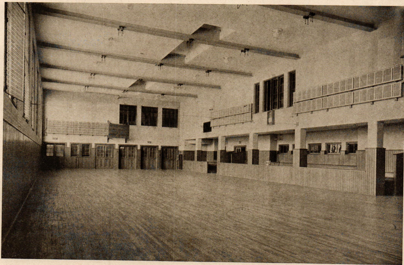
SOUTH JUNIOR HIGH SCHOOL, WALTHAM, MASS. A COMBINED SCHOOL AND COMMUNITY BUILDING KILHAM, HOPKINS & GREELEY, ARCHITECTS
