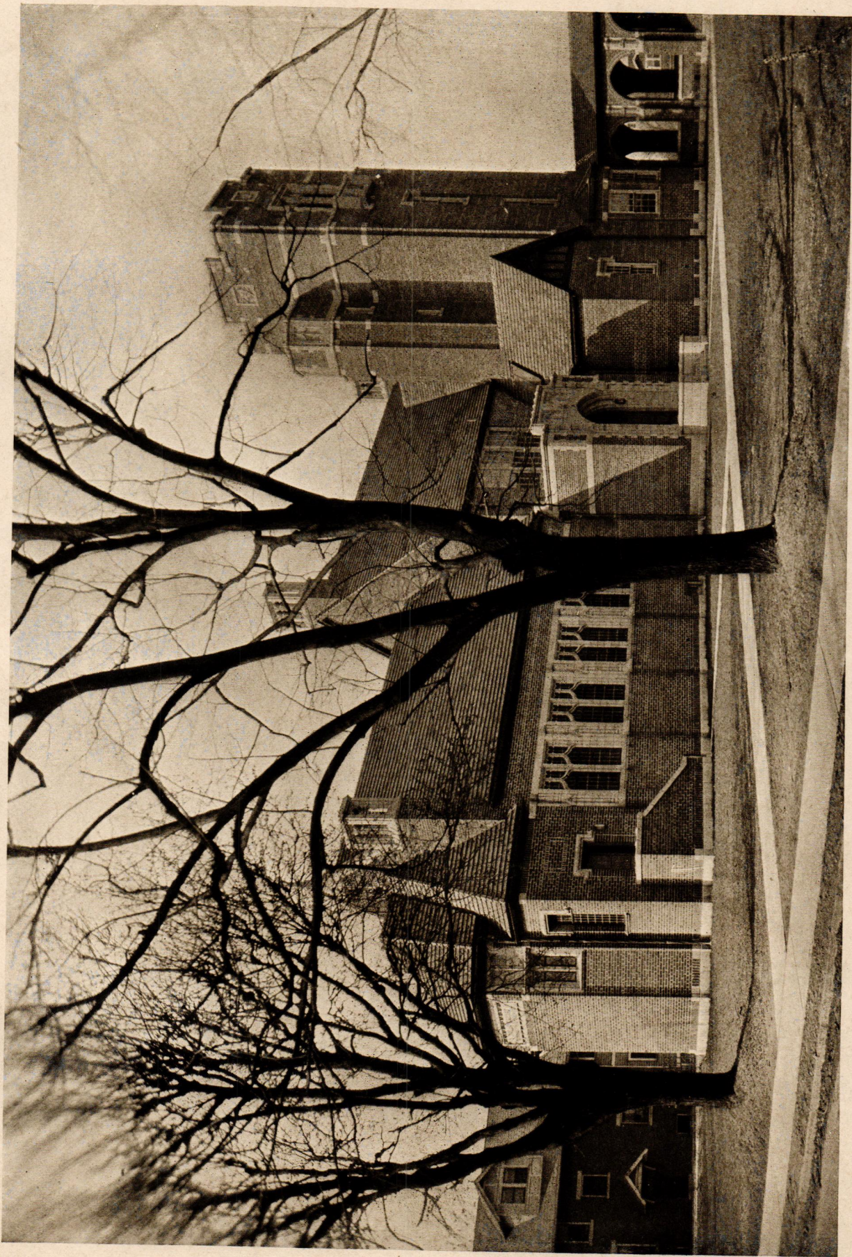
DIVINITY GROUP, CAPITAL UNIVERSITY, BEXLEY, OHIO PERKINS, FELLOWS & HAMILTON, ARCHITECTS
