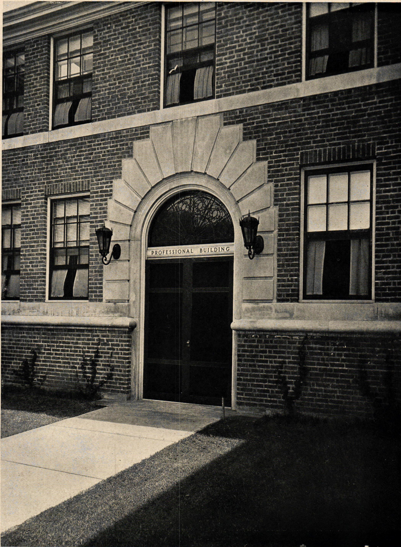
PROFESSIONAL BUILDING, HEMPSTEAD, L. I., N. Y. W. F. McCULLOCH AND GODWIN & SULLIVANT, ARCHITECTS
