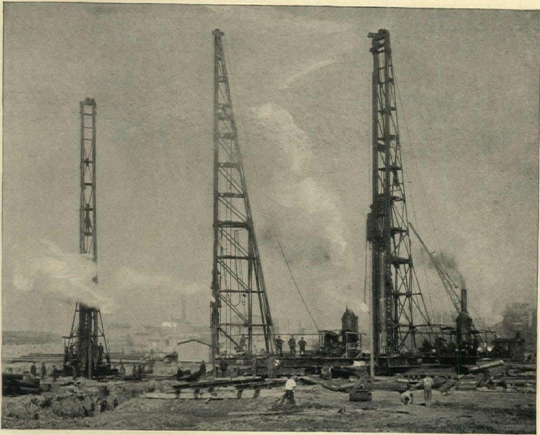
RAYMOND Composite (<sup>Wood</sup>/<sub>Concrete</sub>) Piles not only join timber to concrete in such a way that the transverse strength at any section approximates that of the wood pile . . . . they accomplish this result by a method that permits inspection and checking of each step.
